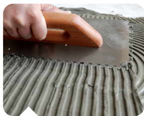
Trowel thinset mortar
