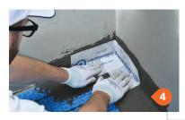
Fix PROBAND 150/250 tape to the same type of adhesive used for tiling following the perimeter joint. Inside and outside corners can be cut from PROBAND 150/250 tape, but pre-cut corners (PRBI and PRBE) are also available on page 19. Using a flat trowel apply strong and even pressure along PROBAND 150/250 to ensure sealing.
