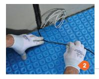
Begin the installation at the thermostat location, ensuring that the heating cable(s) cold lead reaches the thermostat jbox with 6" of slack, and the cable hot/cold splice joint is installed in the membrane where it will be fully embedded in modified thinset or self leveler
