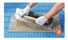
Apply the thin set to the back of the tiles with a notched trowel and lay them on the layer of thin set previously applied. Occasionally remove and check some tiles, to ensure full back coverage.
