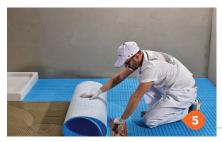
Lay the next sheet of PRODESO HEAT MEMBRANE taking care to align it with the previous one, without overlapping. Align the square reliefs to facilitate the installation of the heating cables.
