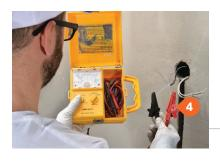
After laying the tiles, repeat all previous tests and record the values obtained in the "Test Log" located on page 38. Ensure all tests are repeated before during and after install.
