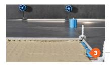
Carefully lay the tiles and press them on the layer of thin set. If a layer of skin has formed on the thin set, remove and apply again.
