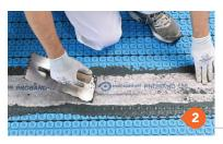
Fix PROBAND 150/250 tape to the same type of adhesive used for tiling following the joint. Using a flat trowel apply strong and even pressure along PROBAND 150/250 to ensure sealing. Smooth over to eliminate bends and folds.
