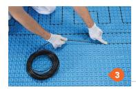
Ensure that the **TRM Heating cable** is evenly spaced across the entire floor. Using the appropriate minimum spacing suggested by TRM, located on page 36.
