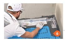
Fix PROBAND 150/250 tape to the same type of adhesive used for tiling following the perimeter joint.
