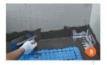
Apply the same type of adhesive used for tiling along the perimeter floor with the flat side of the trowel, to a width of about 4" (100 mm). Particular attention must be paid to fill the cavities of the Prodeso Heat membrane and leaving a thin layer of adhesive on top of the reliefs. Apply the same type of adhesive used for tiling to the perimeter wall with a  $3/16" \times 3/16"$  ( $4 \text{ mm} \times 4 \text{ mm}$ ) notched trowel to a width of about 4" (100 mm).
