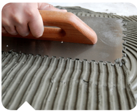
Trowel thinset mortar
