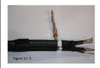
**11.) Figure 11-3**: Slide uninsulated crimp (K) over braid to within  $\frac{1}{2}$  of heating cable.
