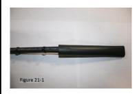
21.) **Figure 21-1**: Slide the heat shrink tube (C) over cables. Place the edge of heat shrink  $\frac{1}{2}$ " past the edge of the mastic strips on each cable.
