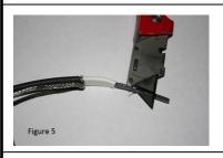
5.) **Figure 5**: Shave off the outer matrix material from conductor with a utility knife. Repeat on opposite side of cable for the second conductor
