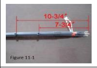
11.) **Figure 11-1**: Carefully align each heating cable on top of one another, pressing mastic strips together. Fasten with a cable tie (D) at  $7 \frac{3}{4}$ " and  $10 \frac{3}{4}$ " from the end of the cable as shown.
