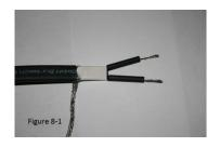
8.) **Figure 8-1**: Slip black heat shrink tubes (G) onto conductors up to the inner jacket
