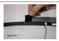
10.) **Figure 10-1/10-2**: Remove paper from mastic strip (E). Wrap a piece of mastic around the outer jacket on each heating cable, 2" down from the end of the outer jacket. (If needed, each mastic strip can be stretched to accommodate thicker types of heating cable)
