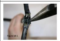
18.) **Figure 18-1**: If the adhesive seals from the heat shrink tubes (F) melt while shrinking cap, pinch again with needle nose pliers as shown.
