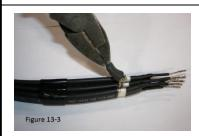
**13.) Figure 13-3/13-4**: Immediately after shrinking, pinch the end of the tube with a pair of pliers and hold until the end stays sealed
