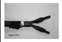
**19.) Figure 19-2/19-3**: Wrap a stretched mastic strip around each of the heat shrink caps as shown. Press mastic strip into itself to ensure a good grip
