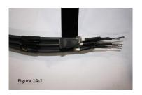
14.) **Figure 14-1/14-2**: Fold the crimped braid back on top of the heating cables. Then wrap the black cloth tape (B), around the crimp and heating cables. Ensure to cover the crimp completely.
