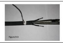
**9.) Figure 9-3**: While tubing is still hot; pinch the end of the tube between the two conductors with needle nose pliers, and hold for 10 seconds to ensure seal.
