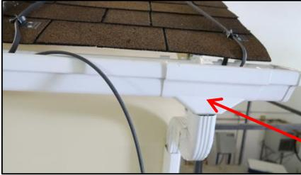
**Figure 1:** Determine the layout of your heating cables and plan out locations where you will be installing your downspout hangers based on where gutters are located, where abrasive transitions are located and/or where cables are to be held down in a gutter
