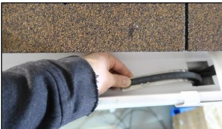
**Figure 5.1:** Position the hanger where it is required and affix cables to the bracket by tightening UV rated zip ties through the pre-drilled holes and around the heating cable
