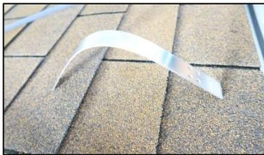
**Figure 3:** Bend the bracket at approximately a 90 degree angle, being careful not to create a sharp bend in the hanger that could potentially cause damage to the heating cable.
