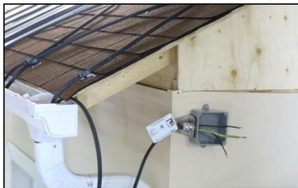
**Figure 9:** Tie into the junction box ensuring the cable is terminated with a drip loop to prevent water run off migrating into the junction box. Connect the Heating cables to the control or GFEP protected circuit.
