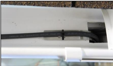
**Figure 7:** Cut off any excess zip tie and ensure bracket is in the proper completed position
