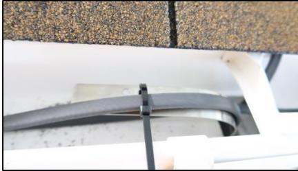
**Figure 5.2:** Position the hanger where it is required and affix cables to the bracket by tightening UV rated zip ties through the pre-drilled holes and around the heating cable
