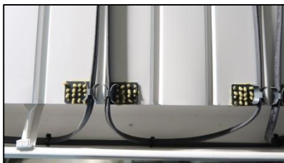
Figure 9: If the roof is a metal seamed roof, ensure that cables are zip tied together using UV rated zip ties at the bottom of each seam, which will ensure cable stability and maximize system performance.
