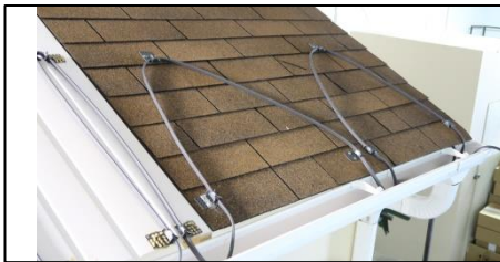
Figure 7: Utilize pliers to fasten the clamps around the heating cable to hold the cable in place.
