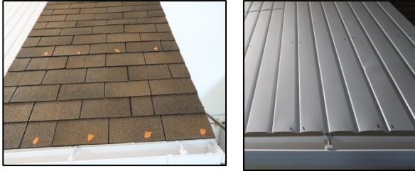
Figure 1: Determine the layout of your heating cables and mark out locations where you will be installing your roof clips.
