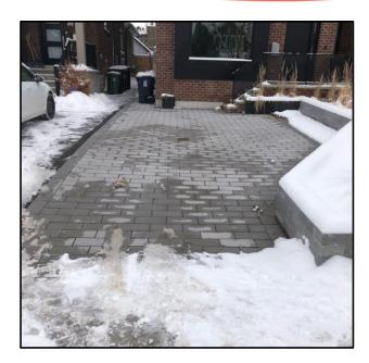
Be ready for Canadian winters and NEVER SHOVEL AGAIN, with Thermal Resources Management brand electric SM Snowmelt heating cables. Designed to output at 15 Watts per linear foot when embedded beneath a concrete slab or paver installation, these cables are the ideal solution for exterior residential snow melting and ice prevention in driveways, walkways, patios, landings and stairs.
